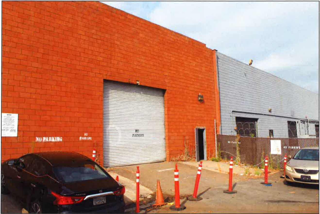
11.0-a Ramp to Entry Door – Bay 2
