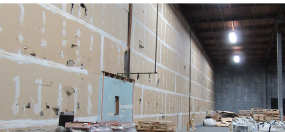
Evaluation of Fire Wall and Sprinkler System
