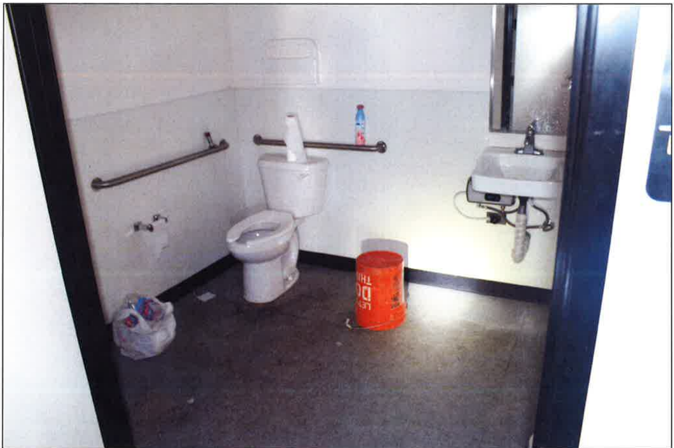
7.2-b Bathroom – Bay 1
