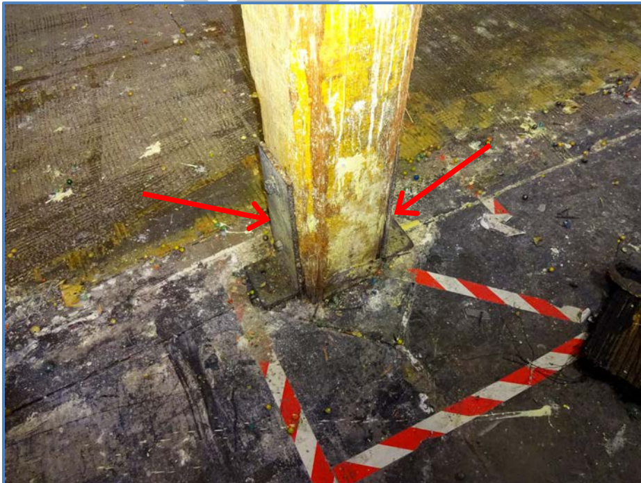
Image 23 – Retrofit Foundation Anchorage
