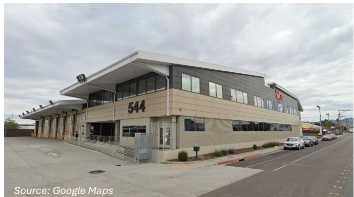
Figure 2-11: ECD Facility and Bus Entrance
