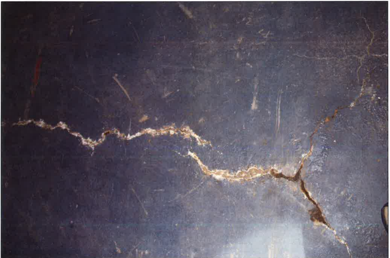
2.3-b Close-up of Previous Photo
