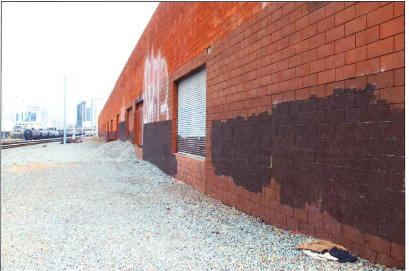
2.0-f West Elevation of Building
