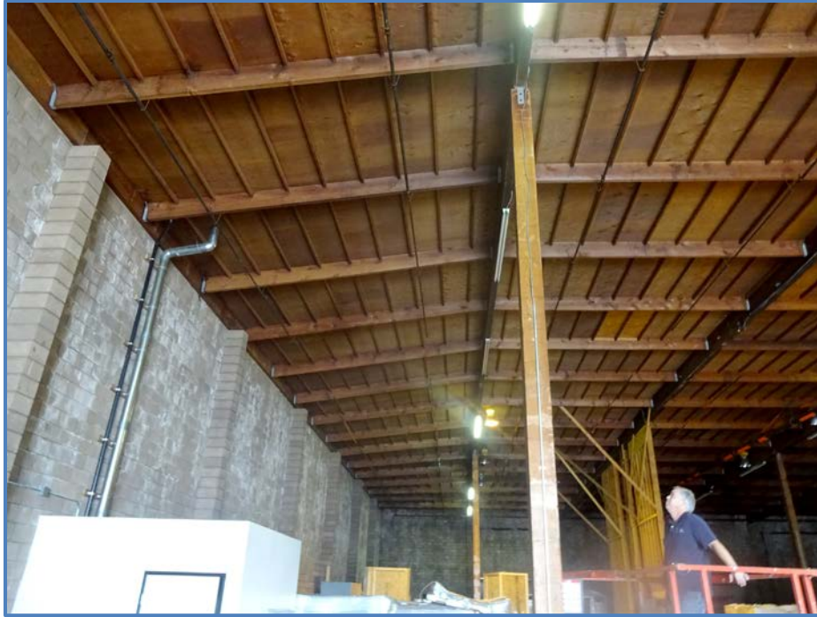
Image 3 – Existing Condition at Short Sides
