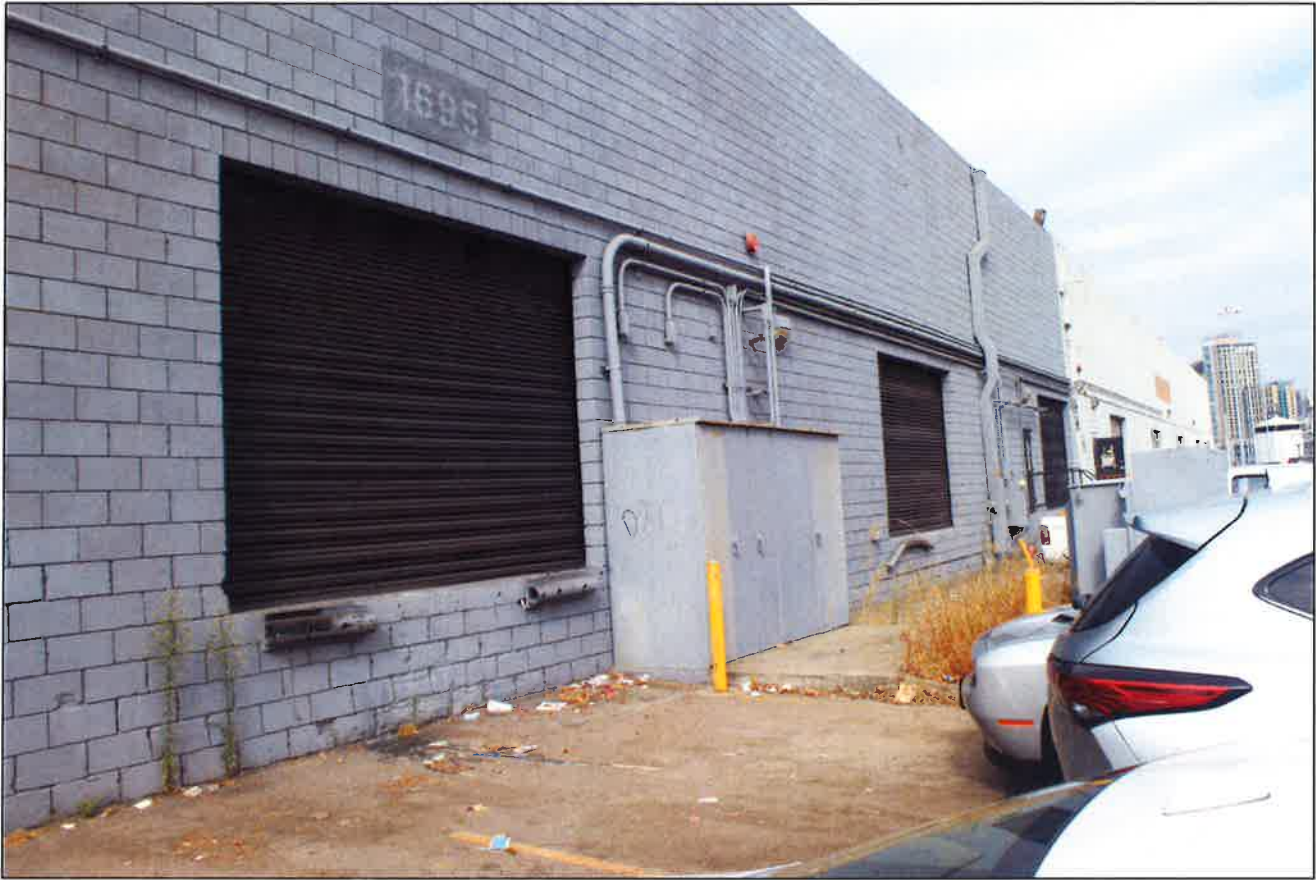
10.3-a East Elevation – Bays 3 and 4
