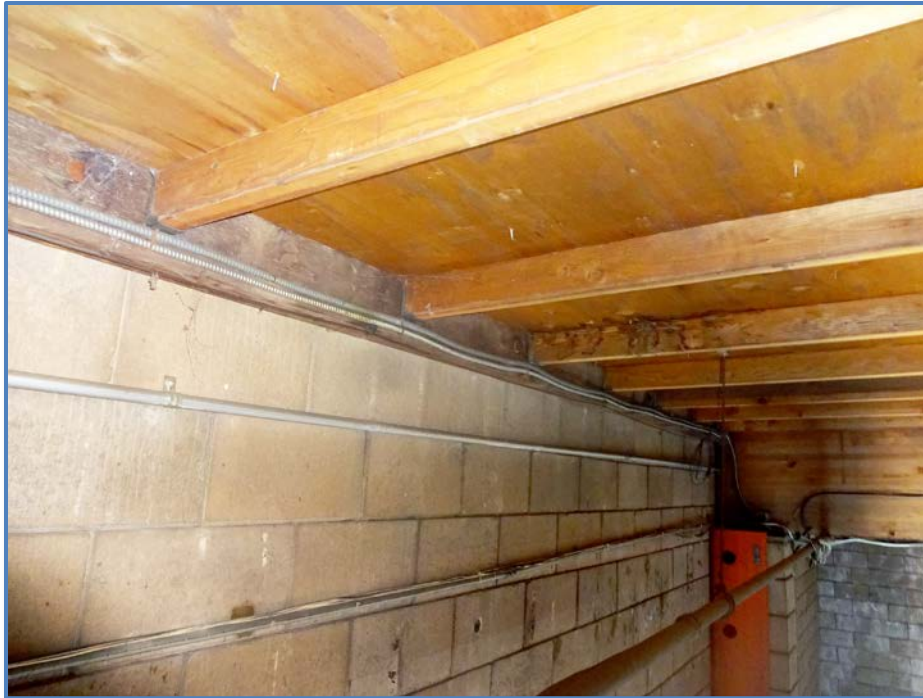
Image 5 – Existing Condition at Long Sides
