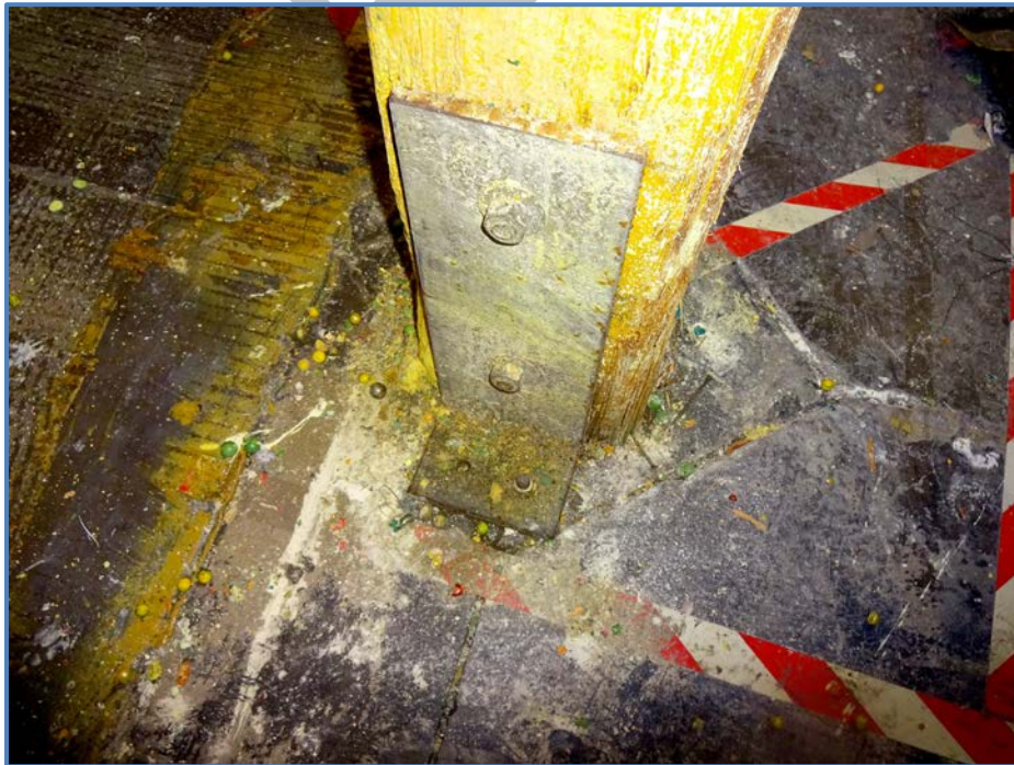
Image 29 – Retrofit Foundation Anchorage
