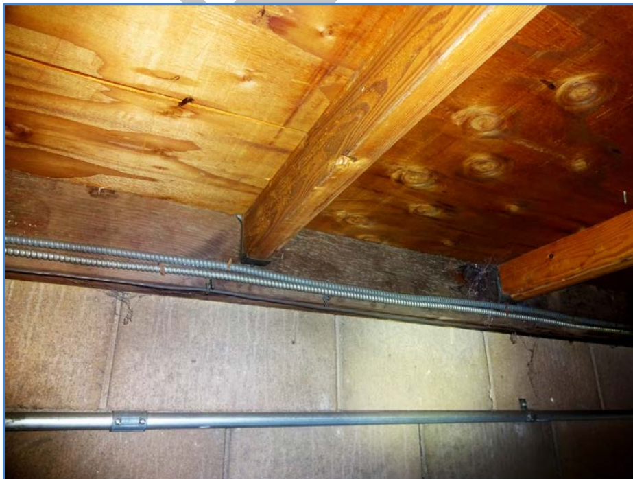
Image 6 – Existing Condition at Long Sides
