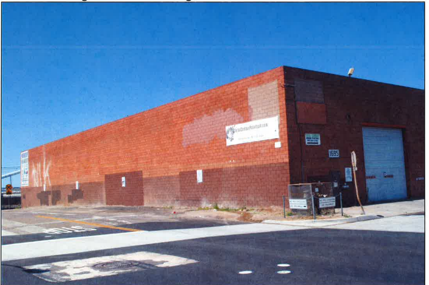
2.0-d Building – From Corner of Sigsbee Street and Main Street – South Elevation
