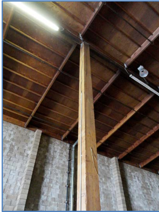
Image 12 - Typical Glulam Column
