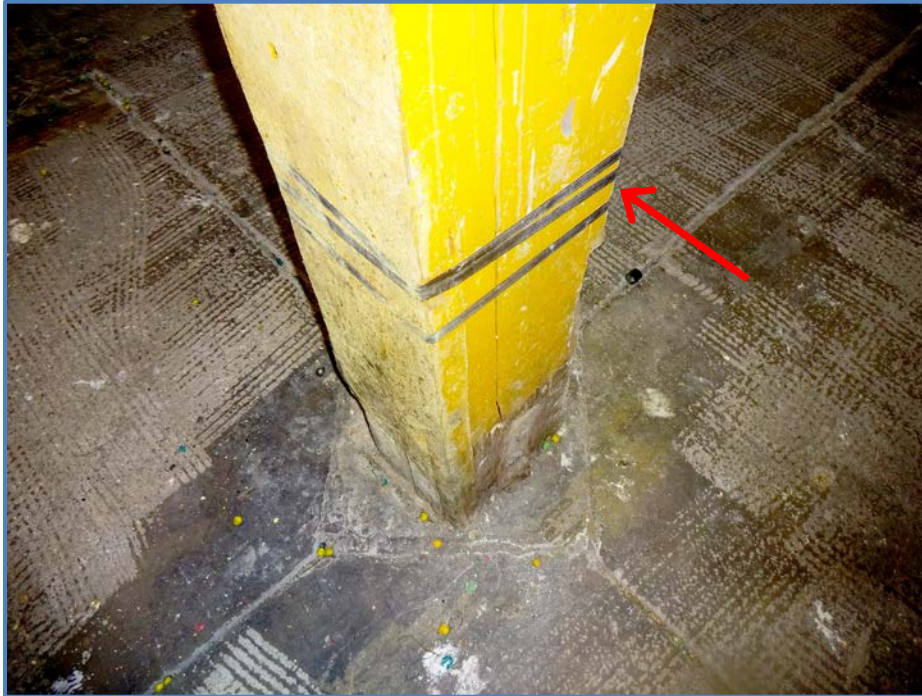
Image 22 – Packing Strap “Repair”
