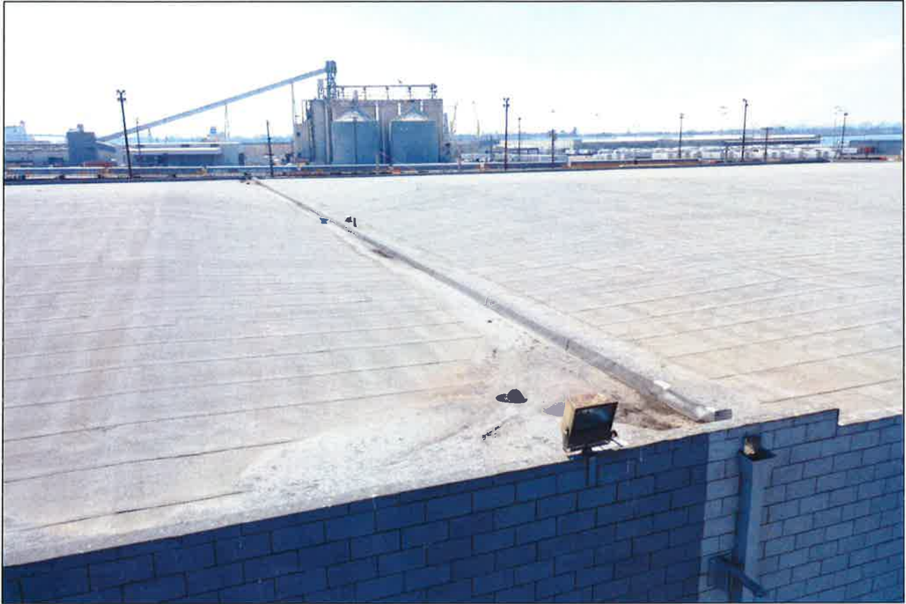
4.0-g Low Curb Between Bays 3 and 4
