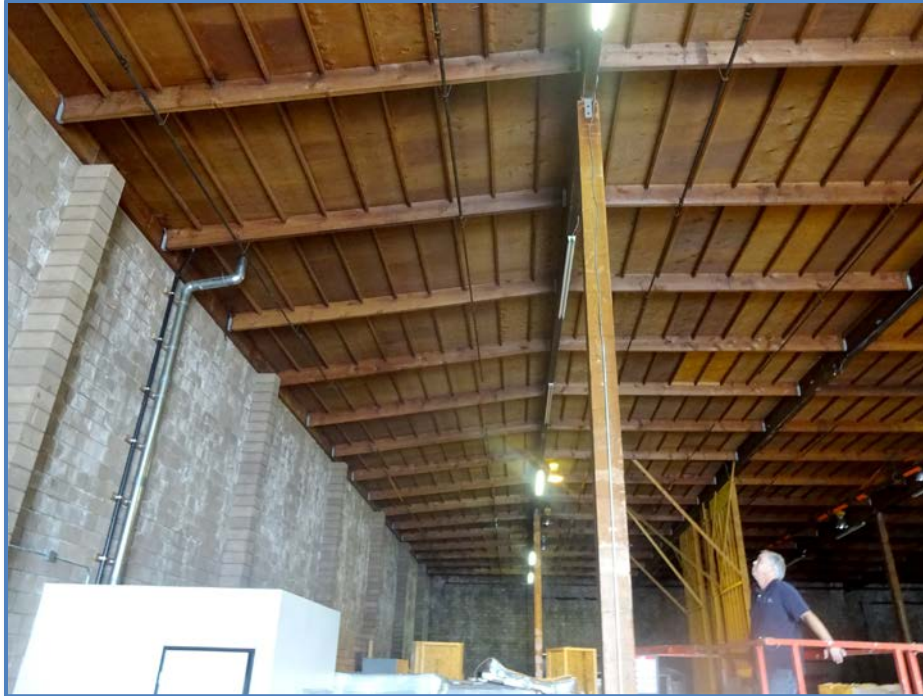
Image 3 – Existing Condition at Short Sides
