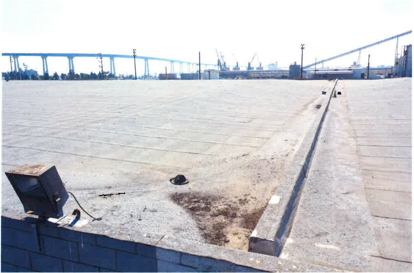
4.1-l Close-up – Low Curb, Vents and Drain
