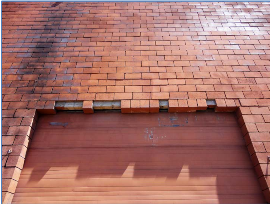
Image 34 – Damaged Lintel
