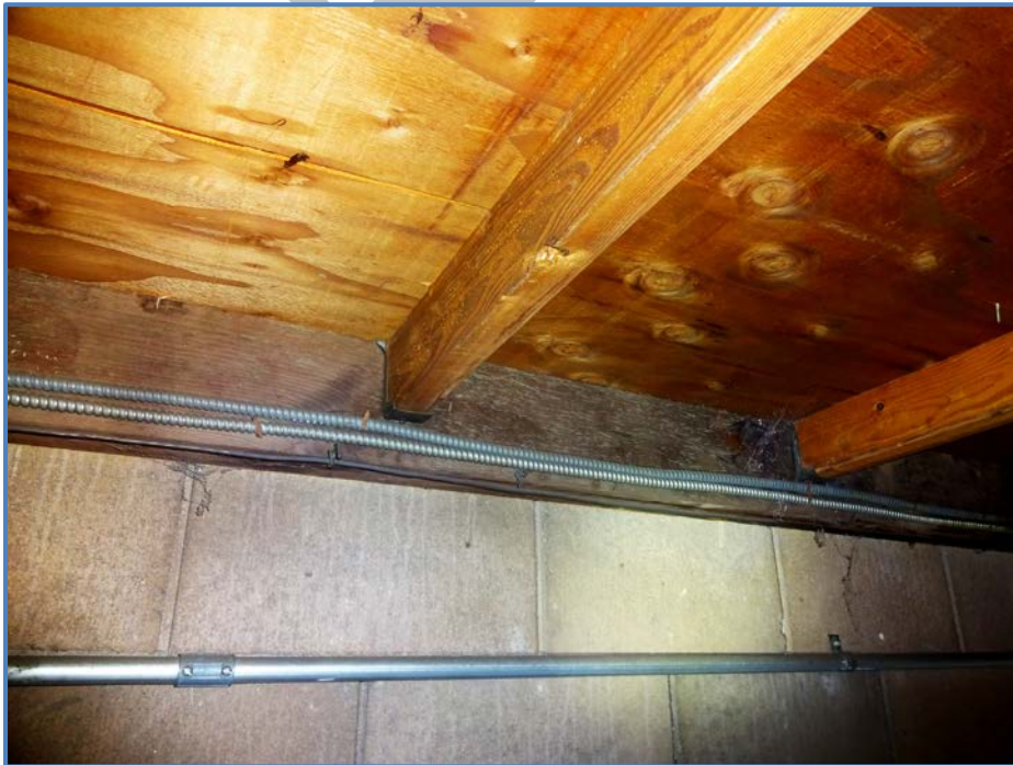
Image 6 – Existing Condition at Long Sides
