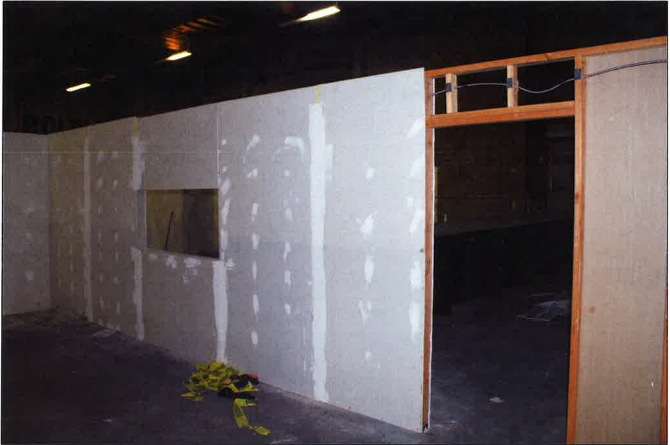
6.3-c Wood Framed Wall – Bay 4
