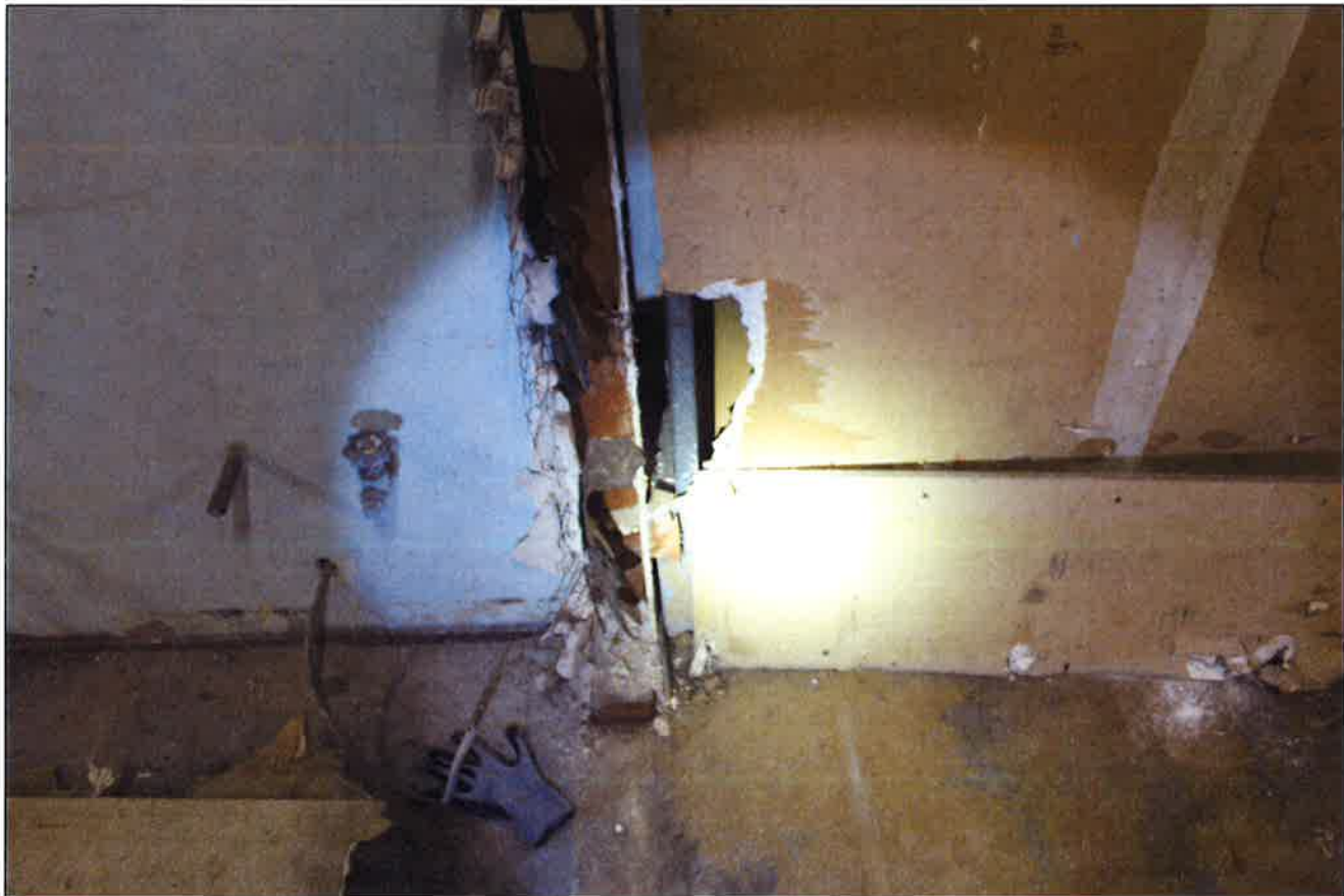
4.0-d Area Separation Wall – Bays 2 and 3
