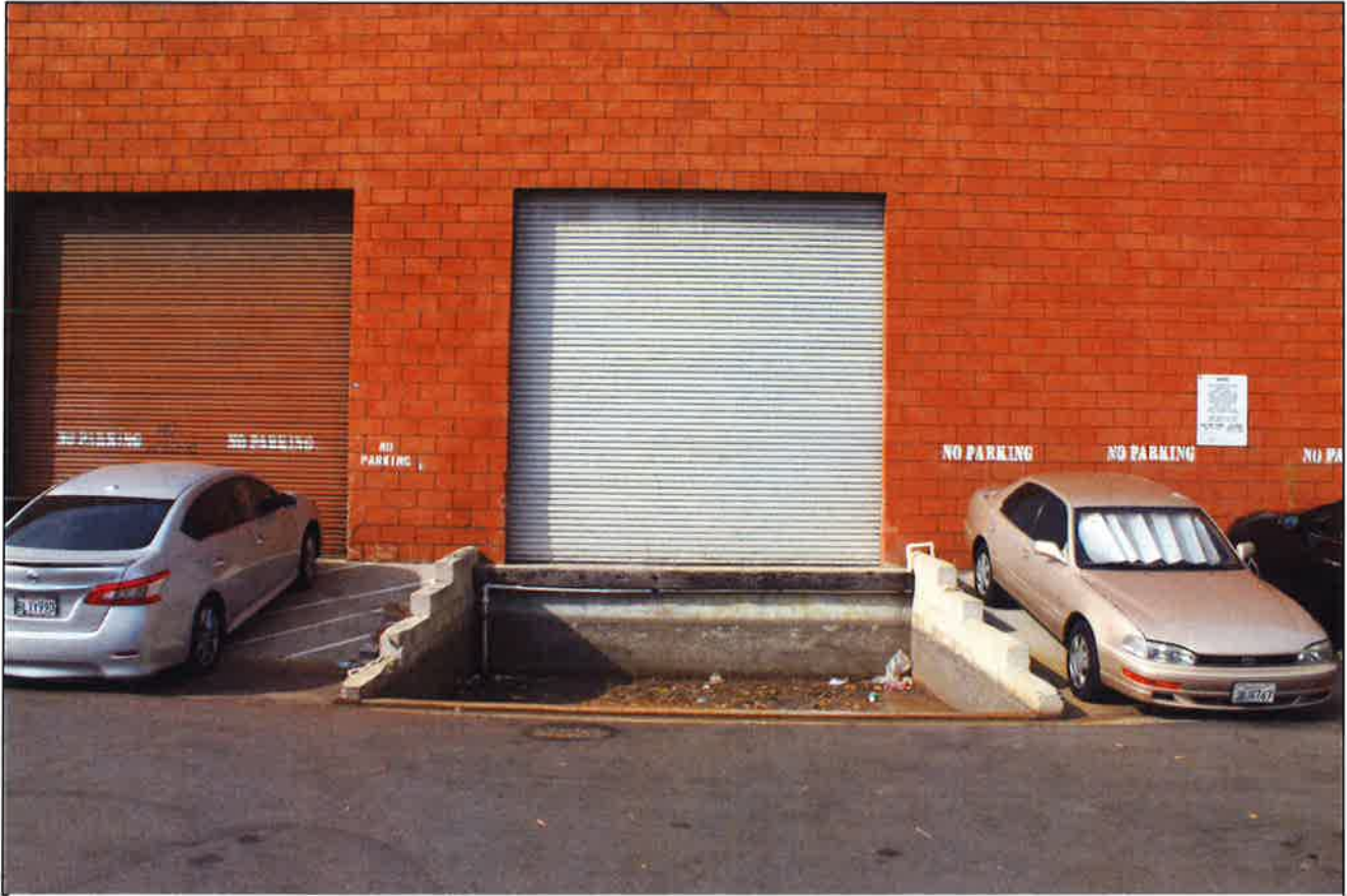
10.2-a Drainage Swale for Parking Lot – Rainwater Fills Truck Ramp and then Continues North in the Swale
