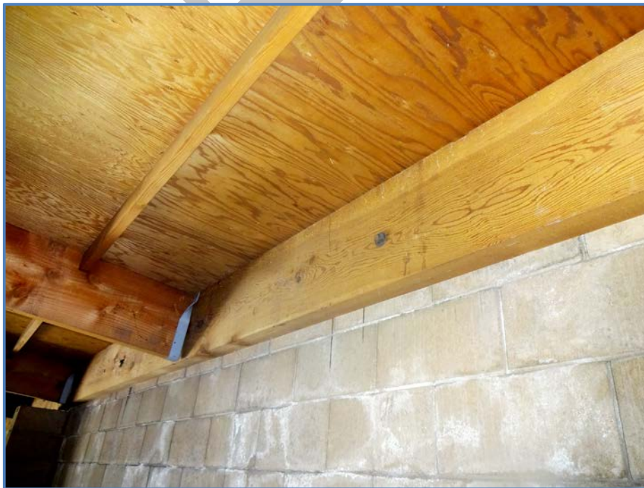
Image 4 – Existing Condition at Short Sides
