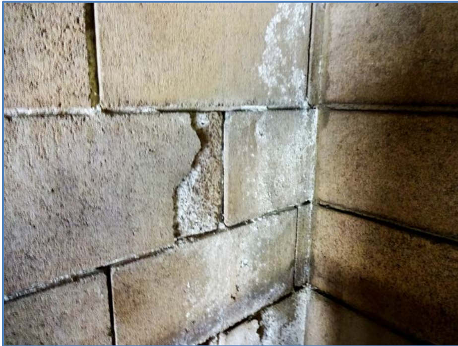
Image 38 – Cracked Block
