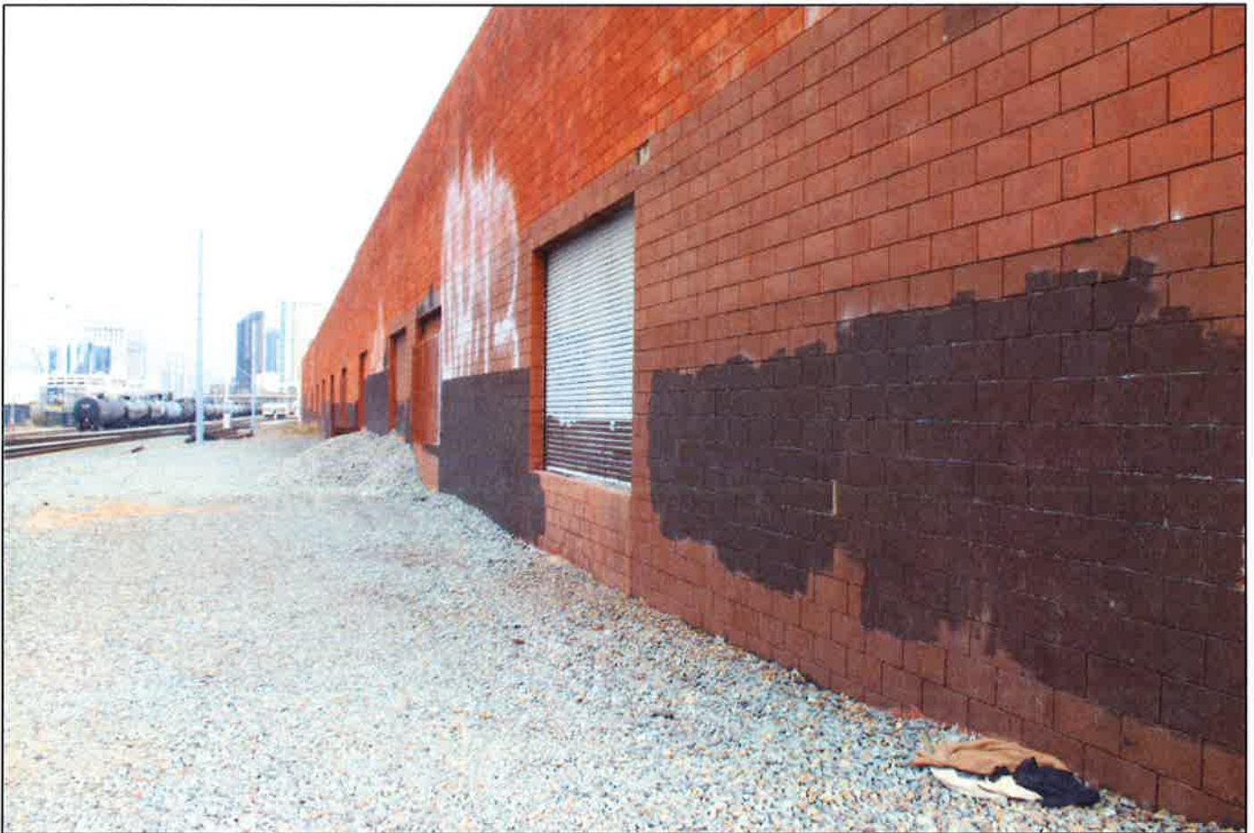
2.0-f West Elevation of Building
