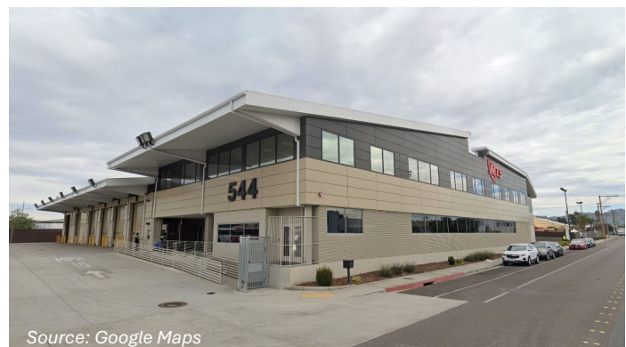
Figure 2-11: ECD Facility and Bus Entrance
