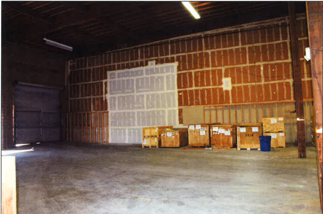
4.0-b Area Separation Wall – Bay 1 and 2
