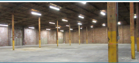
Fire Sprinkler System Evaluation and Egress Requirements
