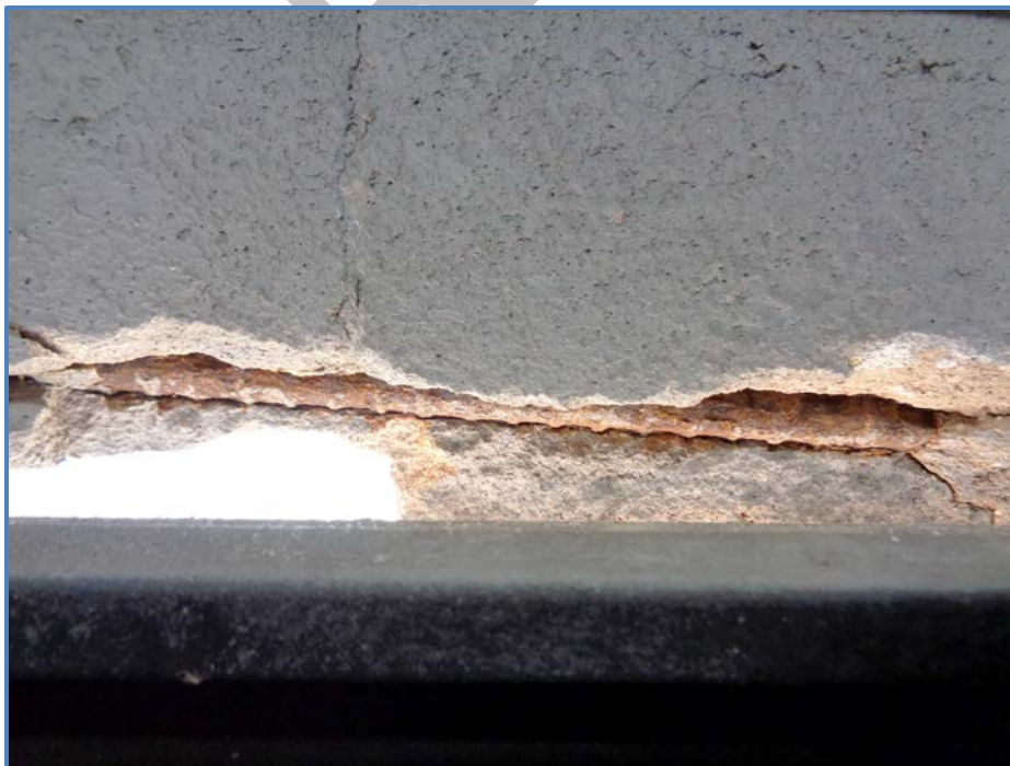
Image 35 – Damaged Lintel
