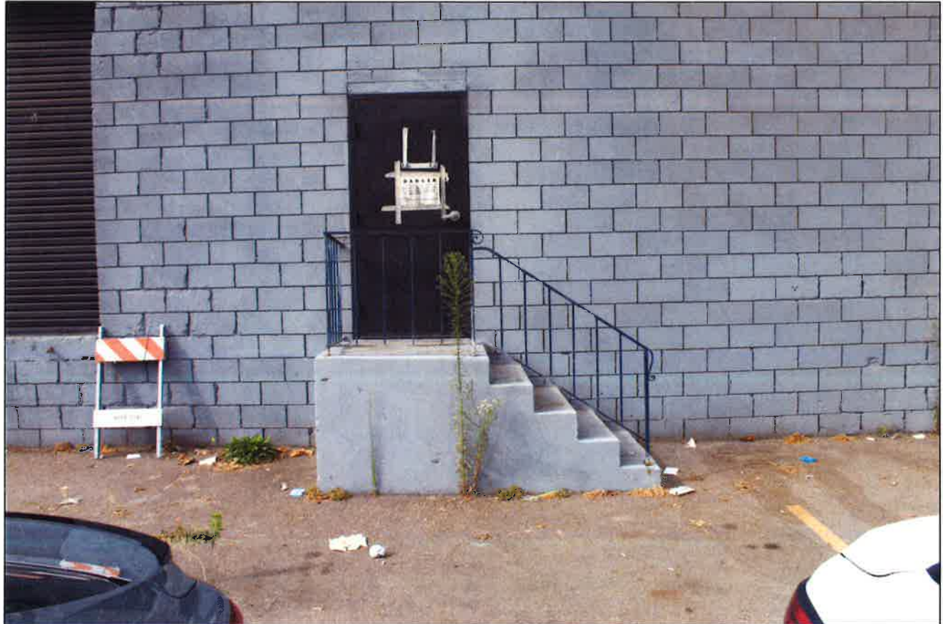
11.0-b Stair to Bay 3
