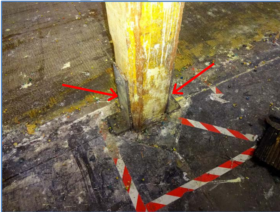
Image 23 – Retrofit Foundation Anchorage
