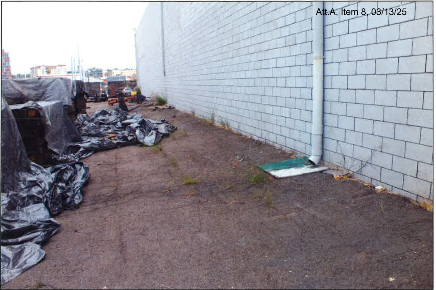
2.0-e North Elevation of Building
