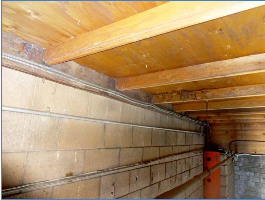
Image 5 – Existing Condition at Long Sides
