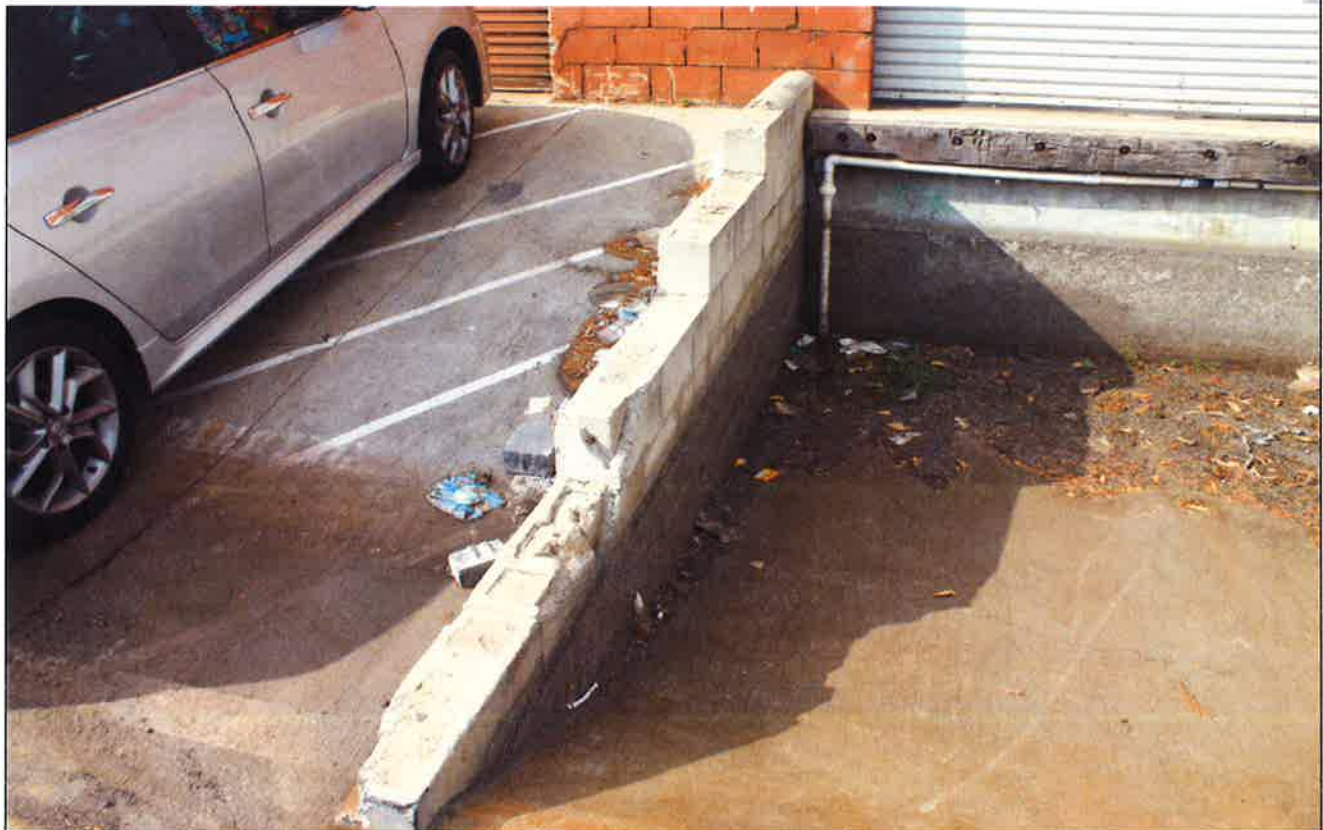
10.2-b Truck Access Ramp
