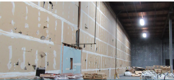
Evaluation of Fire Wall and Sprinkler System
