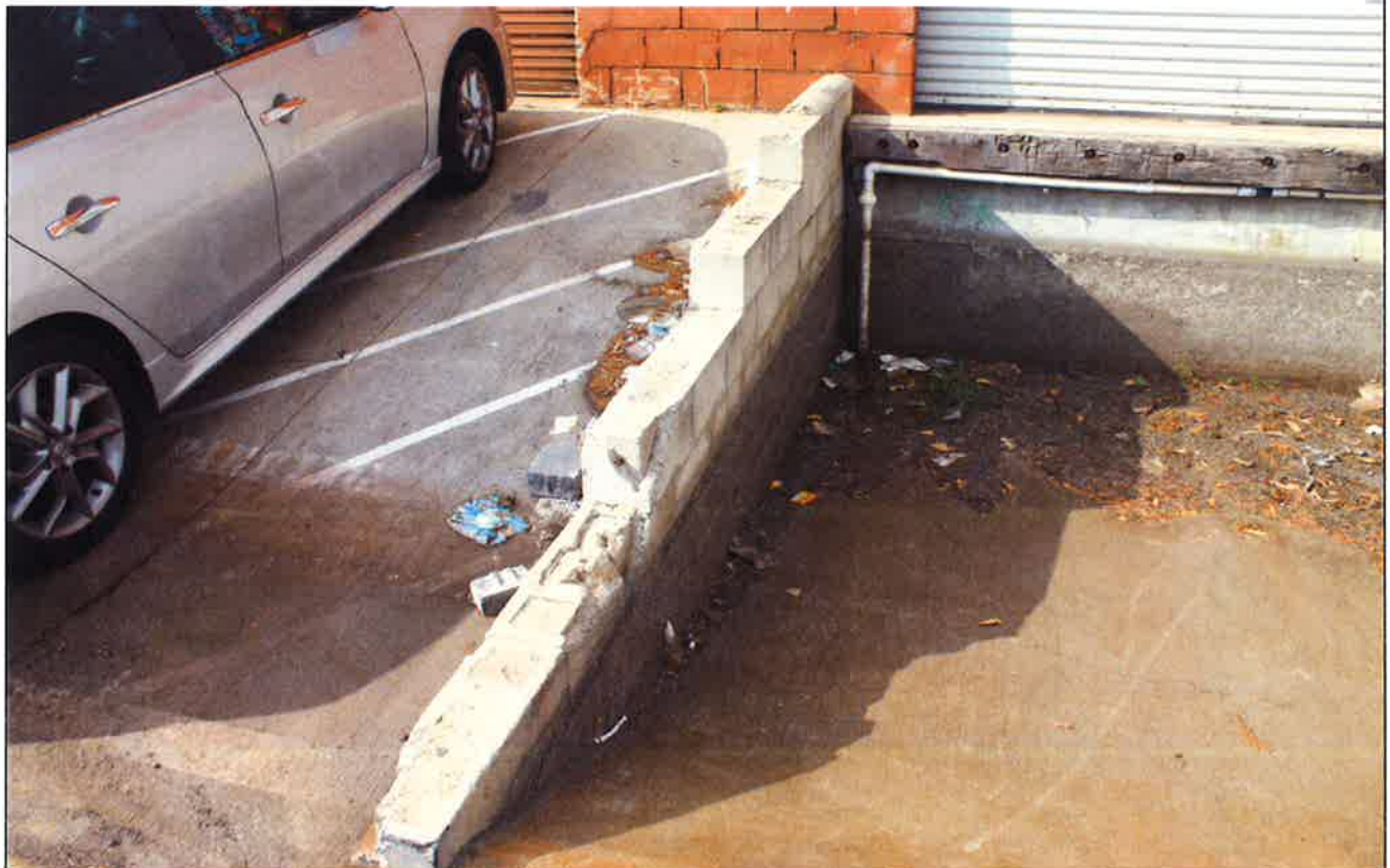
10.2-b Truck Access Ramp
