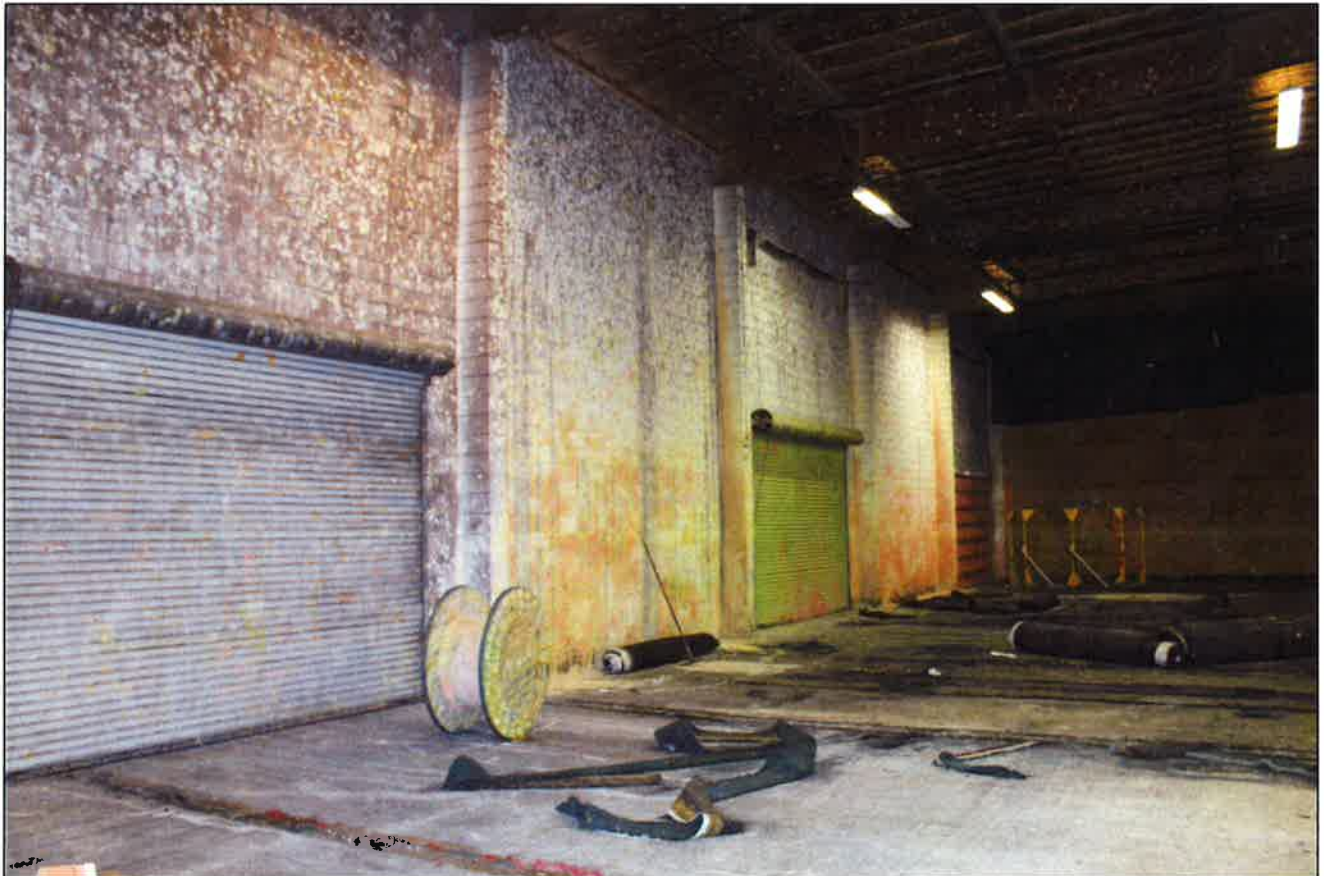
4.0-f CMU Area Separation Wall – Bays 3 and 4
