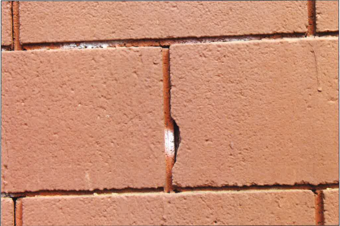
3.1-c Exterior CMU Wall – Open Bead Joints
