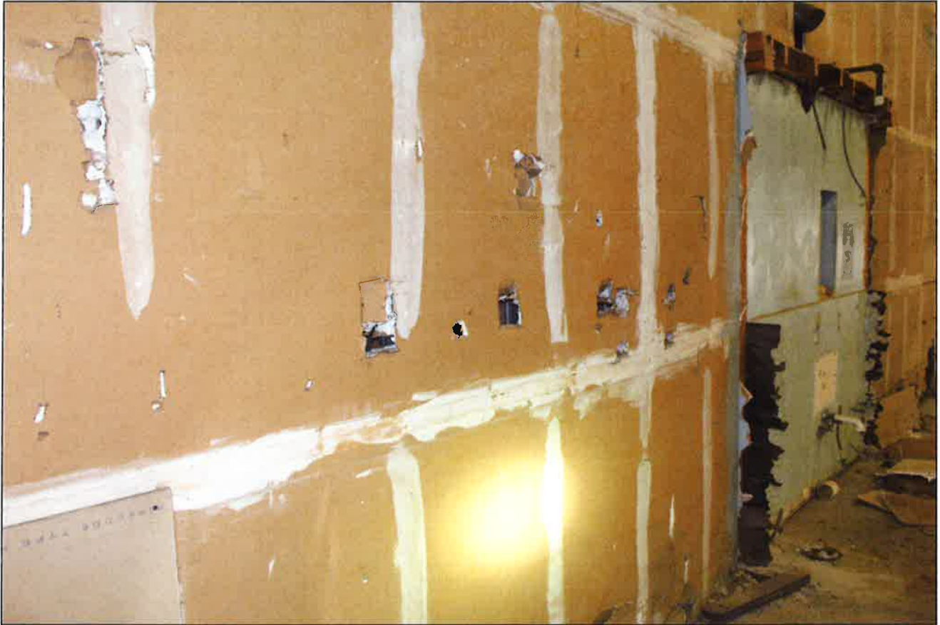
4.0-c Area Separation Wall – Bays 2 and 3
