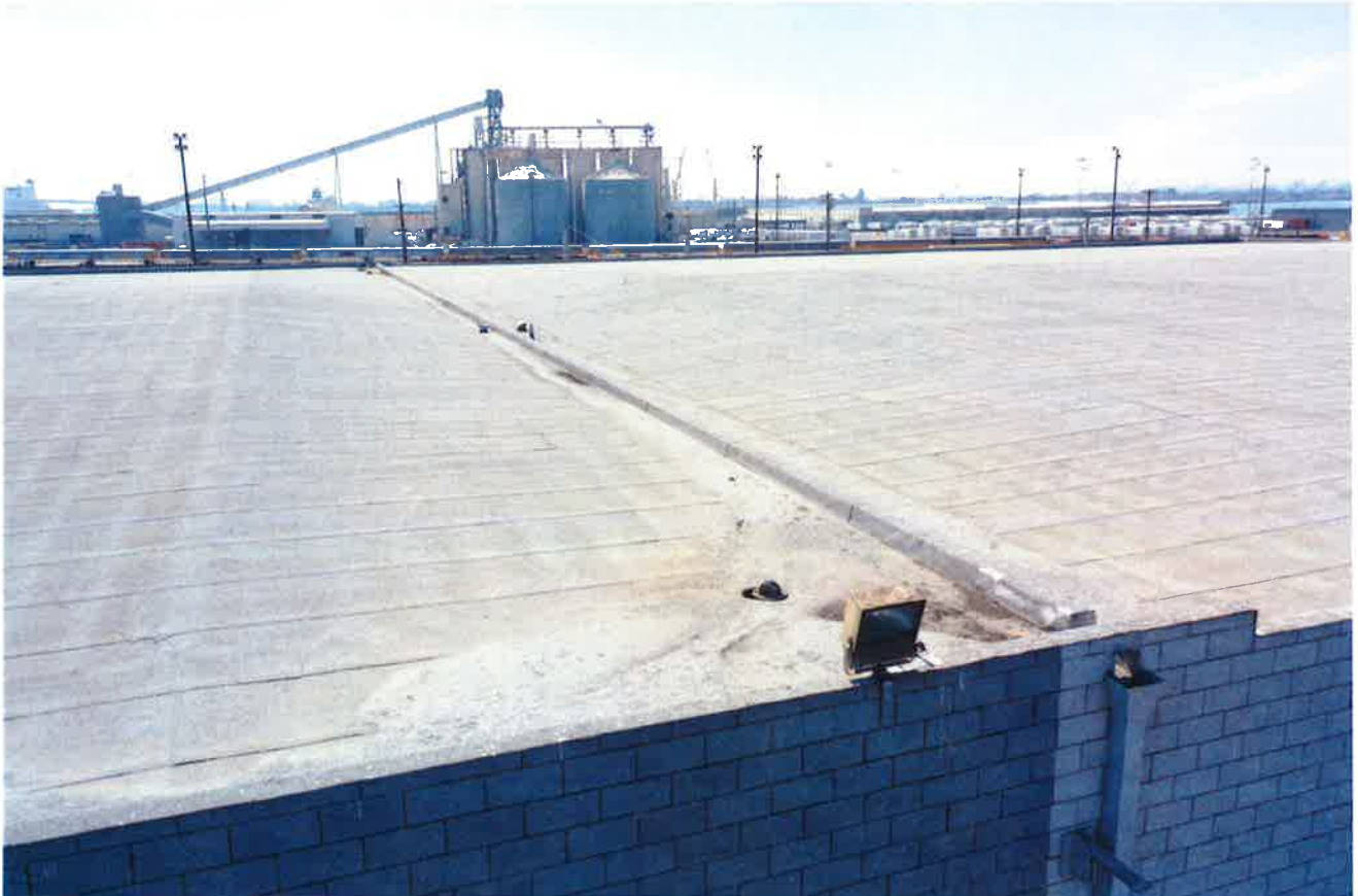
4.1-h Overview of Roof, Low Curb and Scupper
