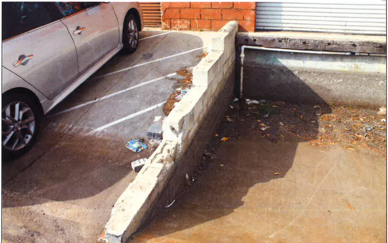
10.2-b Truck Access Ramp
