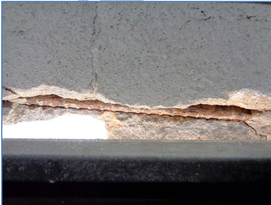
Image 35 – Damaged Lintel
