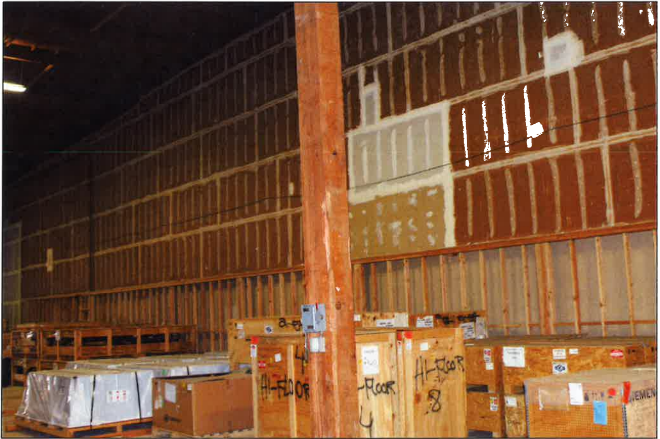
4.0-e Partially Completed Area Separation Wall – Bays 2 and 3
