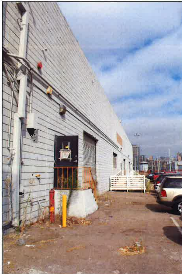
10.3-b East Elevation – Stairs and Ramp – Bay 4
