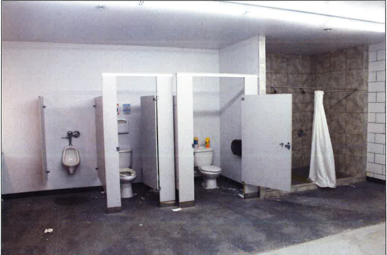
7.2-d Bathroom/ Shower – Bay 3
