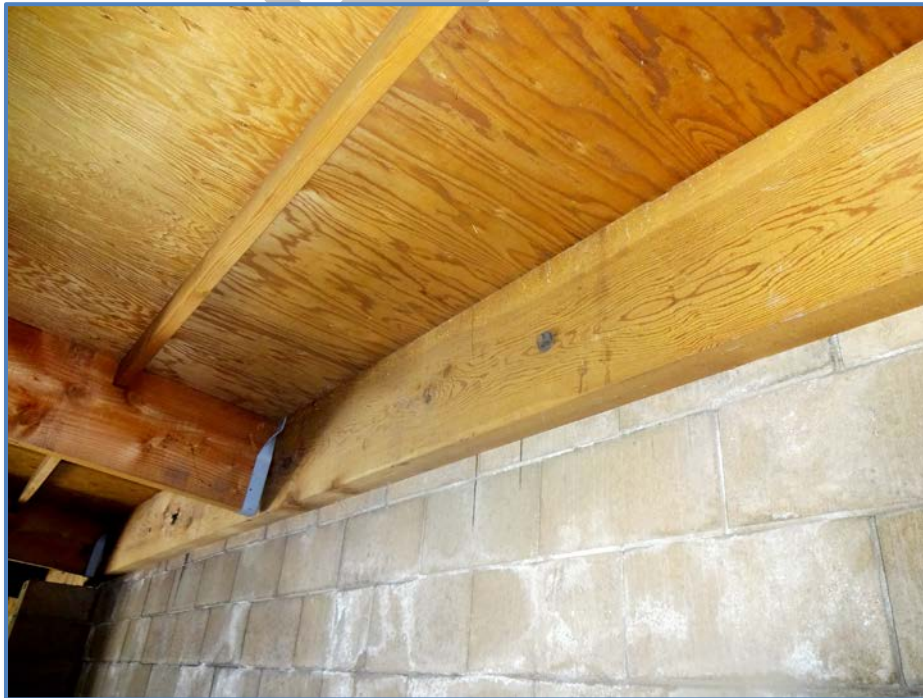
Image 4 – Existing Condition at Short Sides
