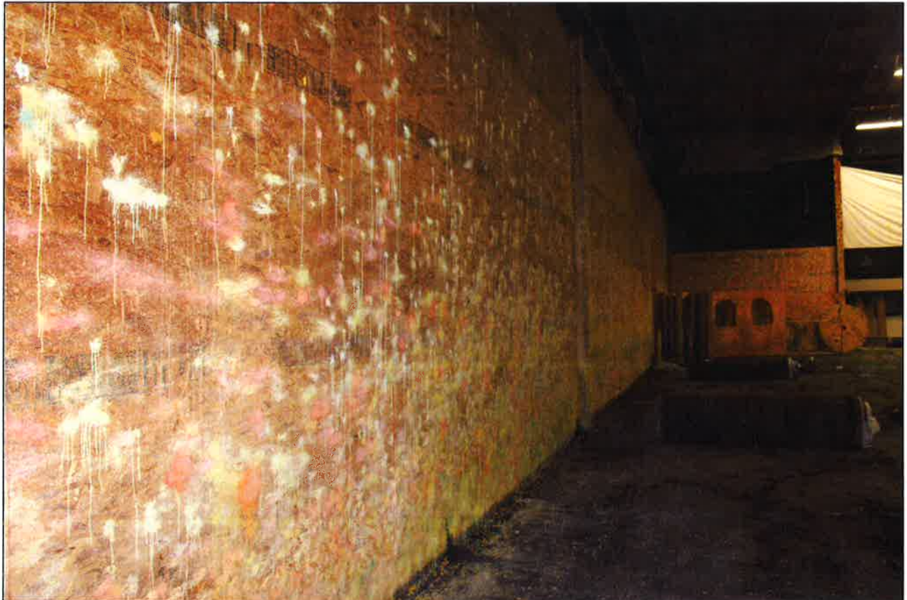
6.3-b Wood Framed Wall – Bay 4
