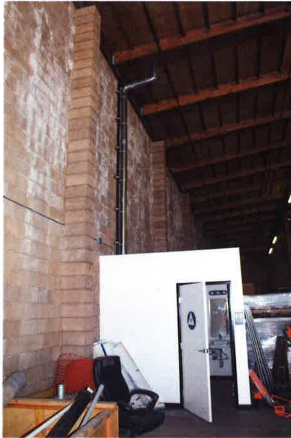
7.2-a Bathroom – Bay 1
