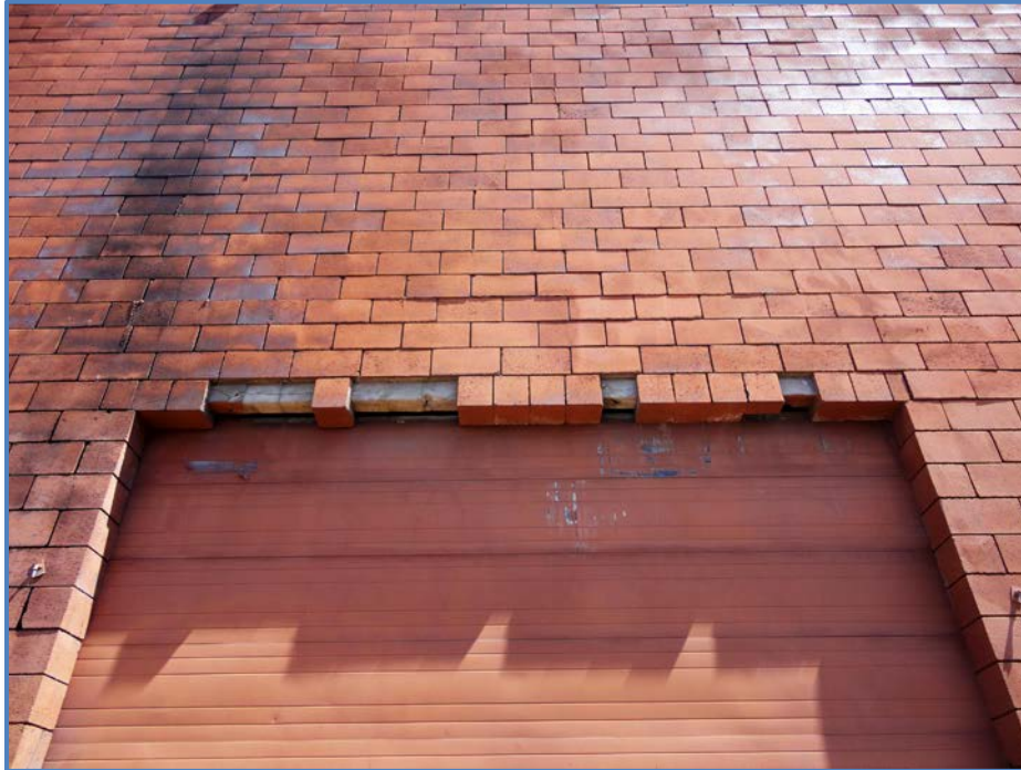
Image 34 – Damaged Lintel
