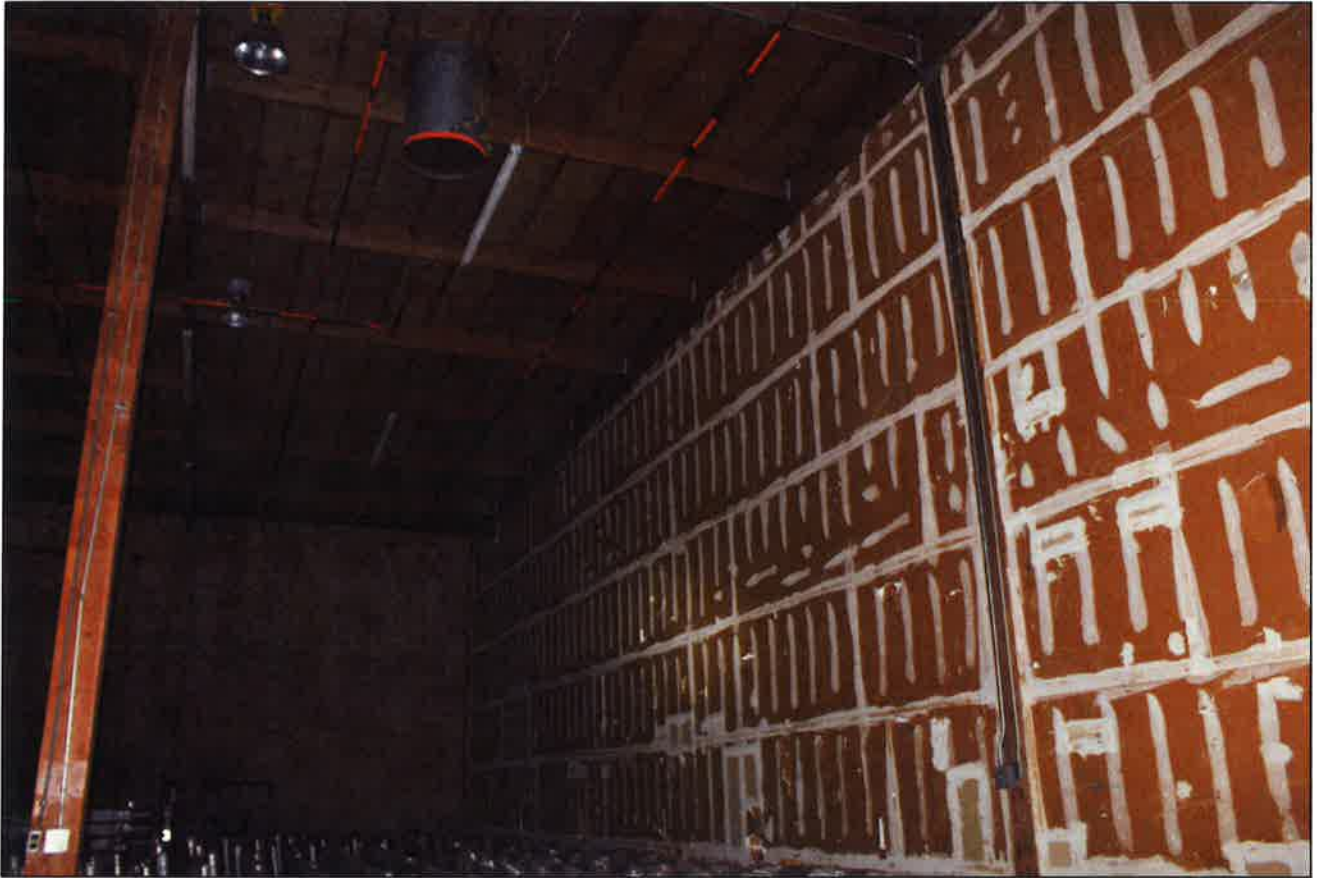
4.0-a Area Separation Wall – Bay 1 and 2
