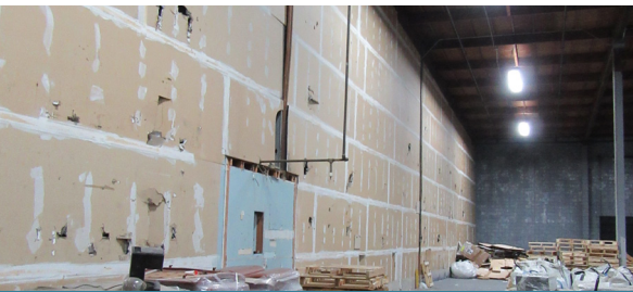
Evaluation of Fire Wall and Sprinkler System
