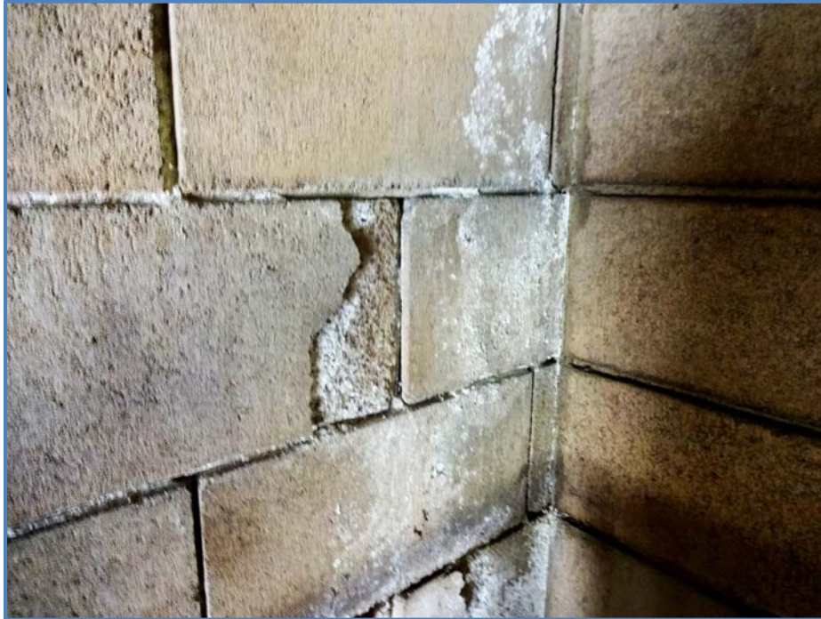
Image 38 – Cracked Block
