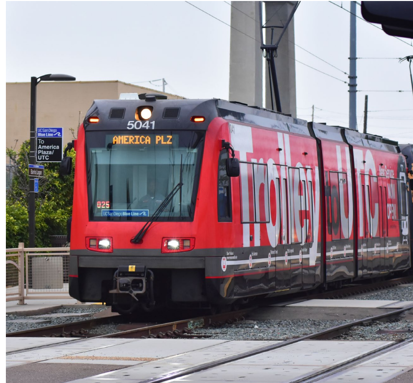
Light Rail Trolley Extension
