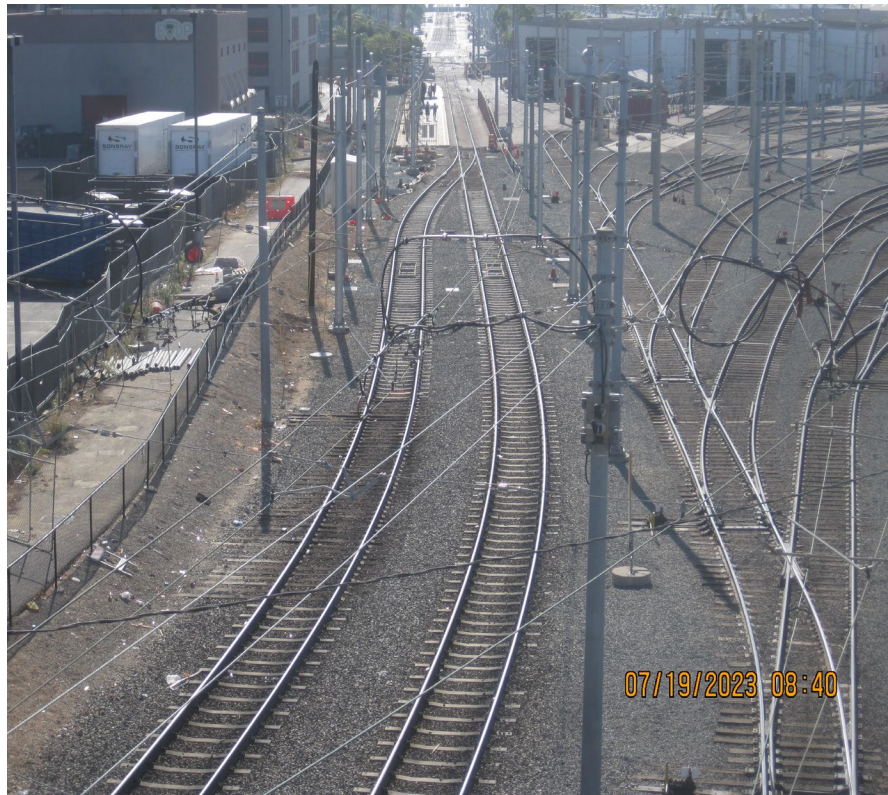
Before: Single Terminal
