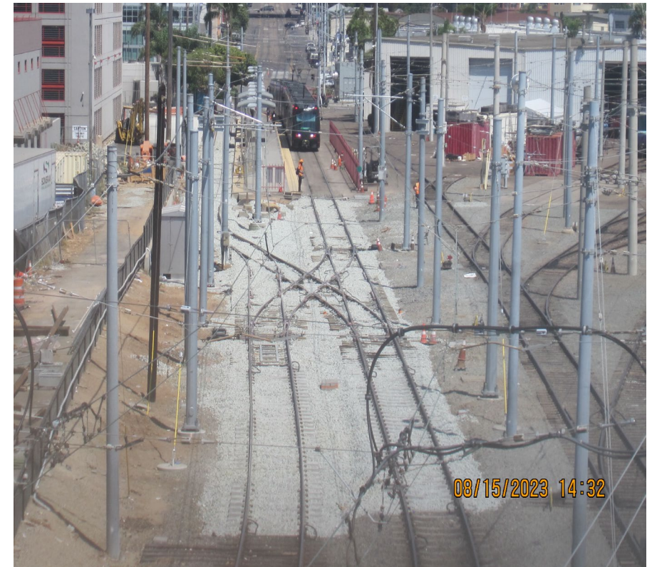
After: Double Terminal
