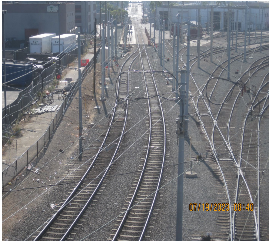
Before: Single Terminal
