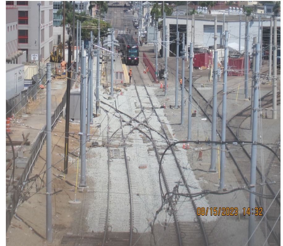
After: Double Terminal
